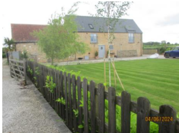
Rear elevation of The Old Dairy
